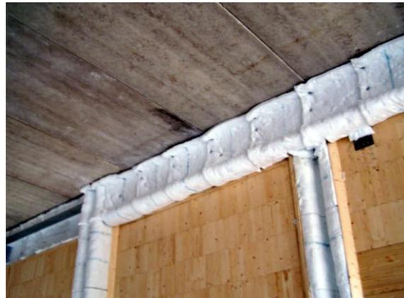
Extensive use was made of two low-biopersistence fibre products chosen for their lack of smoke generation in fire due to the absence of chemical binders used in manufacture. Lightweight fire insulation for the steel structure was provided by the flexible-wrap FireMaster 607 Blanket system, whilst thermal and acoustic insulation was provided by Superwool Plus Blanket, a high thermal-efficiency, A1 reaction to fire classified, flexible, blanket with approximately 25% lower thermal conductivity.
