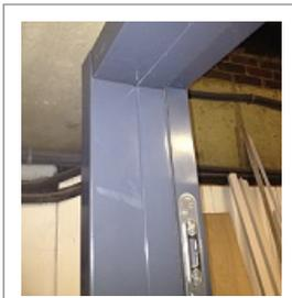
**London Fire Solutions** (LFS) has developed a Steel Frame Armour system, designed to cover existing timber door frames with a recessed housing for its standard 3-point locking system and fire rated hinges.
