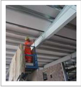
The company says that, unlike traditional water-based intumescent coatings specified to protect structural steelwork, the SC900 series can be applied in a single coat of up to 6.5mm thickness. Reducing application and drying times by over 60% compared to similar systems that require multiple applications, the same 120 minute fire protection is achieved, but allows following works to commence far quicker.
